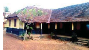
Fig. 2a. Vernacular building
