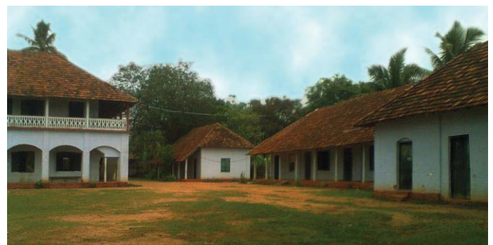
Fig. 3. Single and double storied vernacular school buildings
