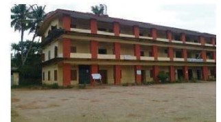
Fig. 2b. Modern building
